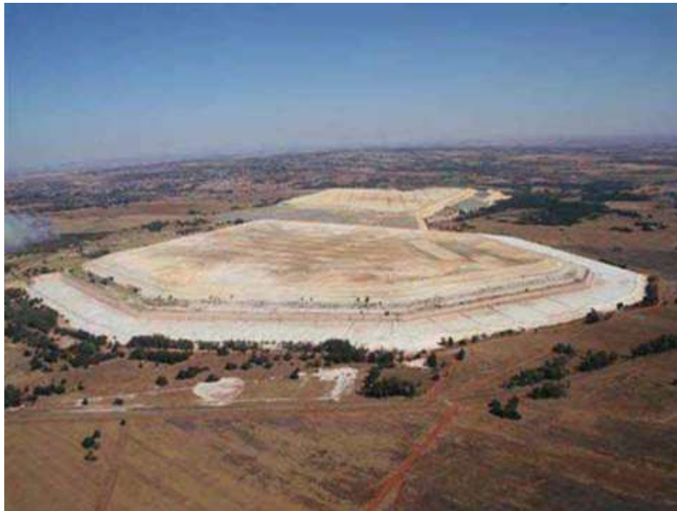
Tailings Storage Facility (West Rand)
