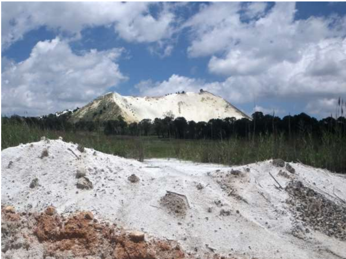
North Sands Dump within the West Rand where the reclamation was not completed due to the low grade of gold in the remainder of the Dump. Note the tailings spillage within a wetland.
